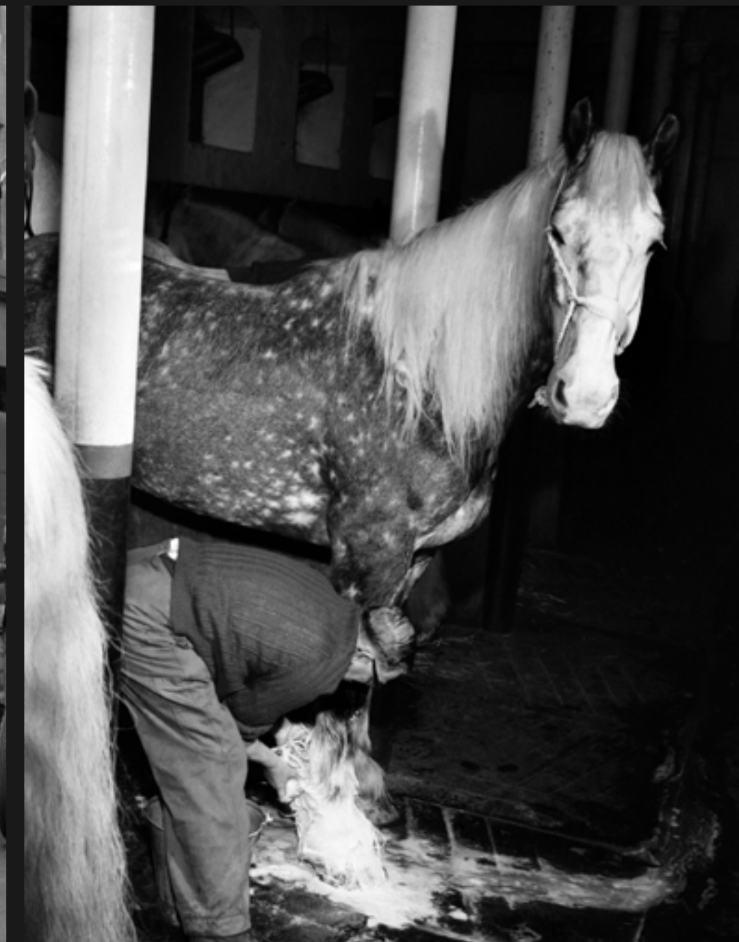
Inside the former stable
